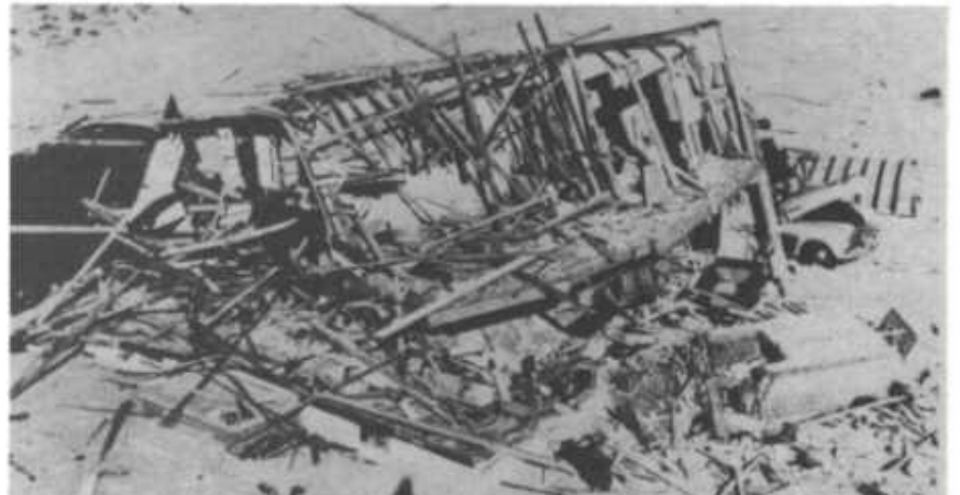
Fig. 7.4. Unburned wreckage of the same two-story, wood-frame house pictured in Fig. 7.1 after being wrecked by the 5-psi blast effects of a small nuclear test explosion.
