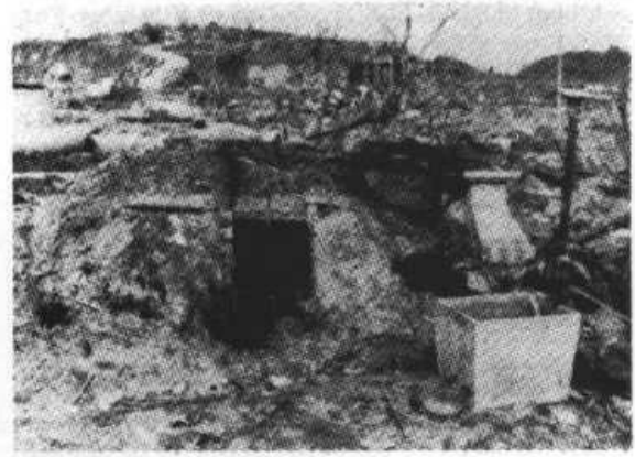
Fig. 1.5. Undamaged earth-covered family shelter in Nagasaki.
