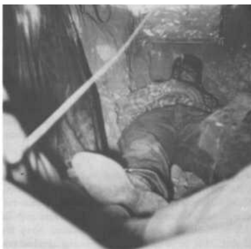
Fig. 6.3. Pulling a Small, Stick-Frame KAP to Keep Temperatures Endurable for Occupants of a Car-Over-Trench Shelter in Warm Weather. Enough air also can be supplied with a small Directional Fan, although more laboriously.
