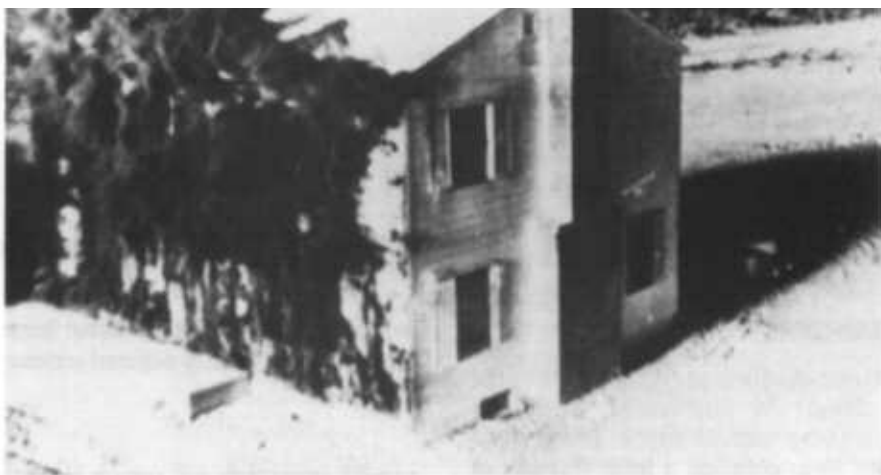
Fig. 7.1. Heat radiation charred the paint on this house, which had been painted white to reflect heat rays. The charring instantaneously produced the smoke. However, precautions had been taken to prevent this typical U.S. house from being destroyed by fire, because the test was made to enable engineers to study the effects of blast, rather than fire. The house was demolished by the 5-psi overpressure blast that struck seconds later, but it did not burn.
